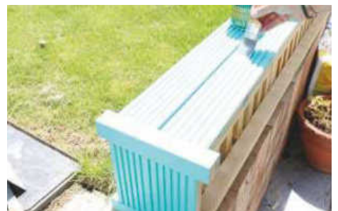
An external top coat is applied to seal the surface, ready for the Pearl Effects
